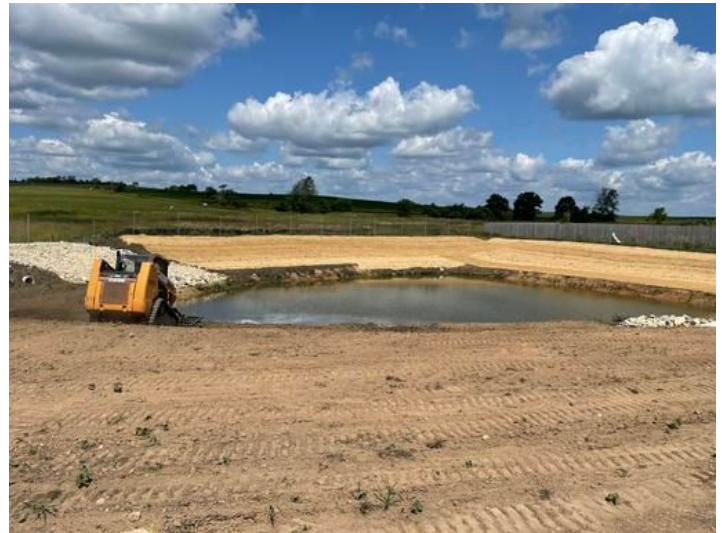
grass seeding the basins Taken on Jul 20, 2023, 11:03 AM CDT Added on Jul 20, 2023, 11:41 AM CDT Added by andrew gordon
